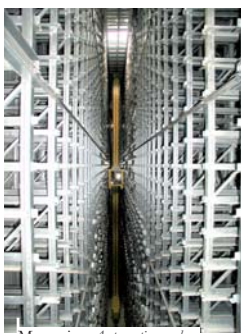
Magazzino Automatic warehouse
